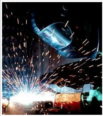
welding in progress
